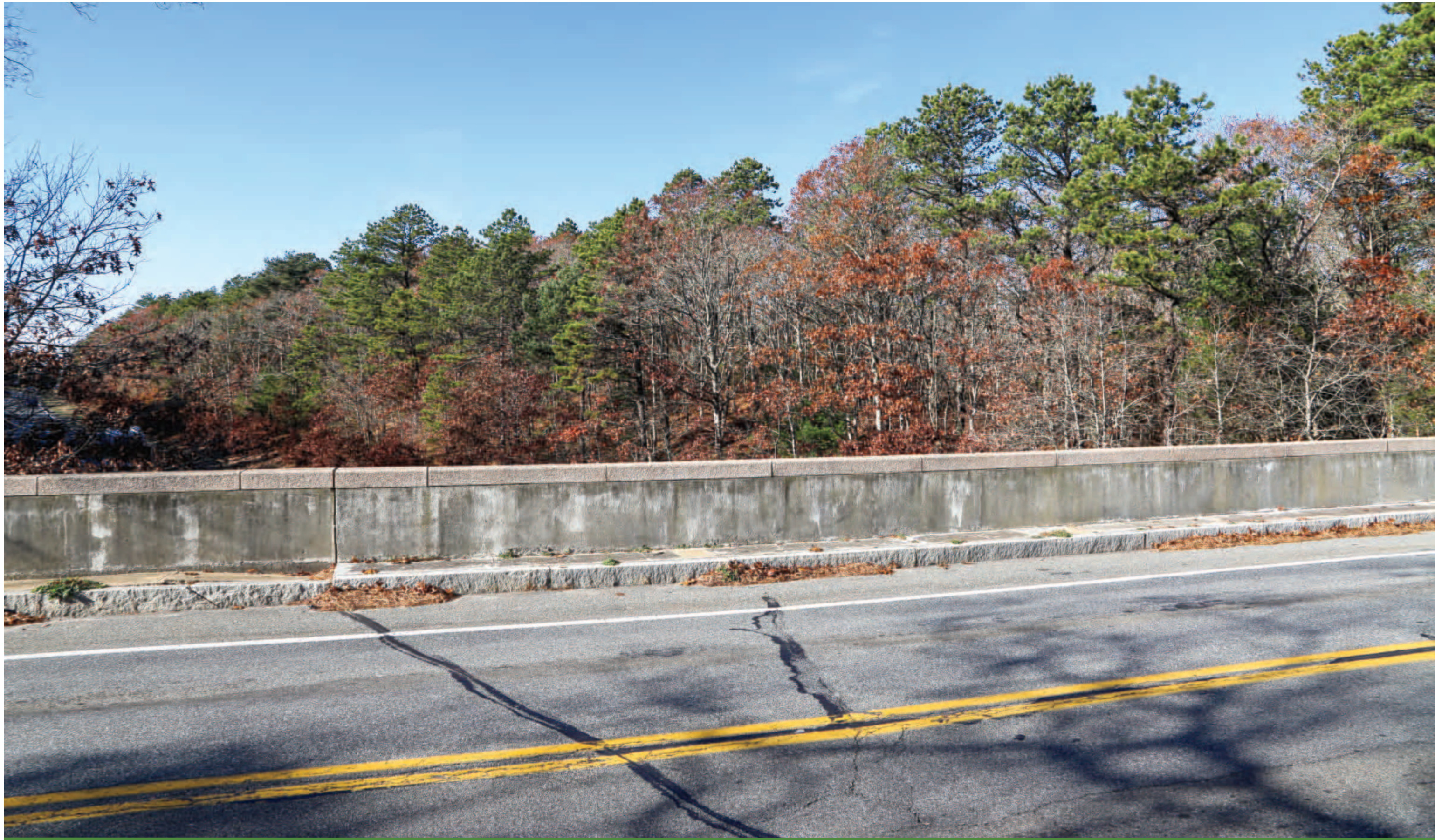
EXISTING CONDITION VIEW Photo 23: Oak Street at U.S. Route 6 Overpass
