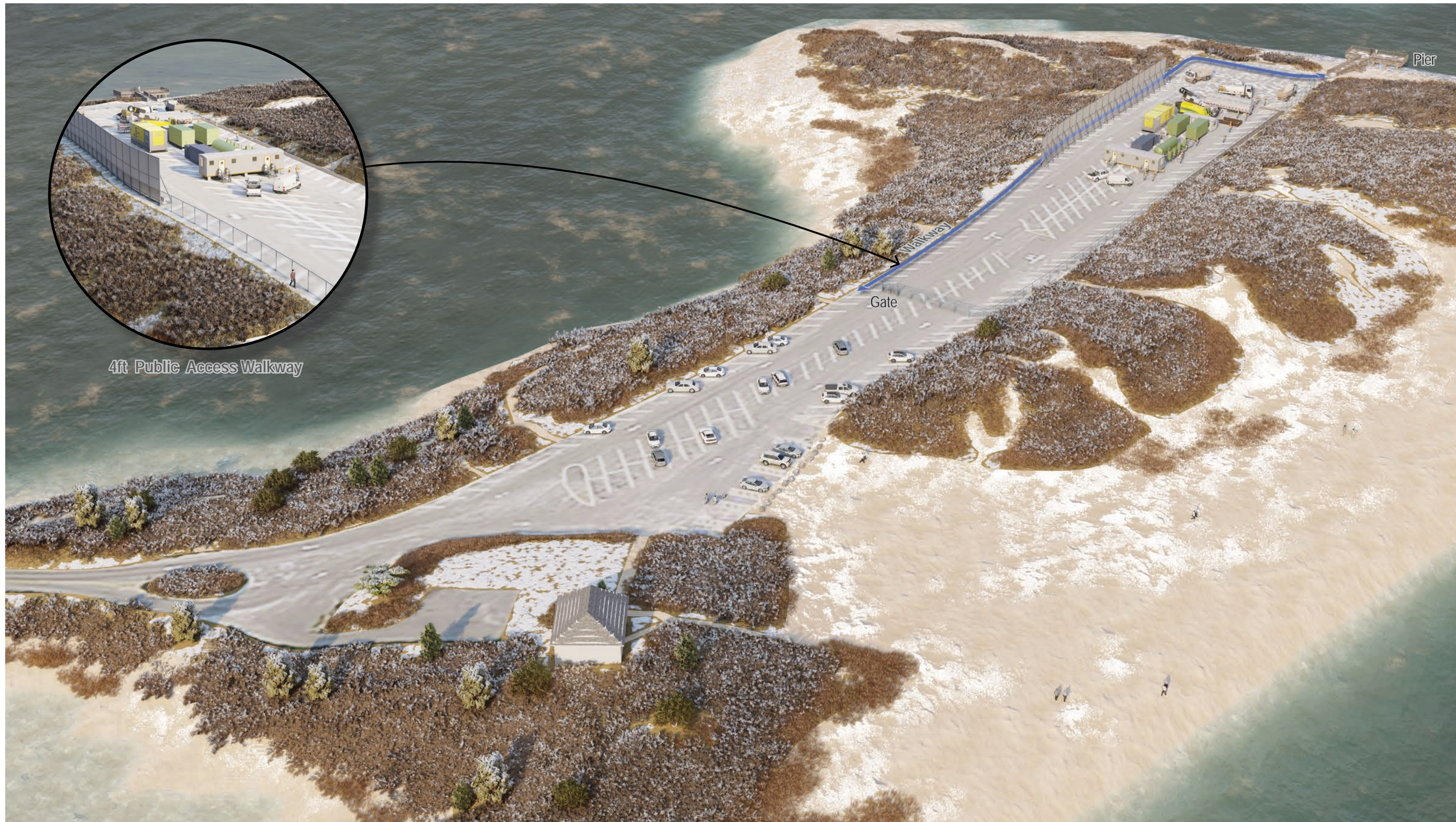
North HDD Construction Staging Construction Season 1
